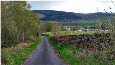
Figure 5. Road width does not meet recommended width for timber haulage
